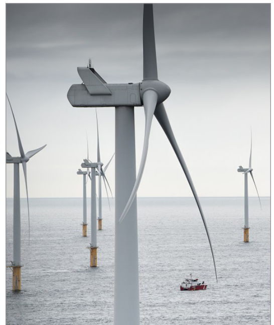
Courtesy of MHI Vestas Offshore Wind
